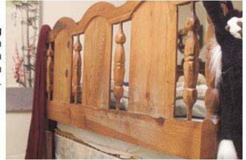
Mold growing on a wooden headboard in a room with high humidity.
